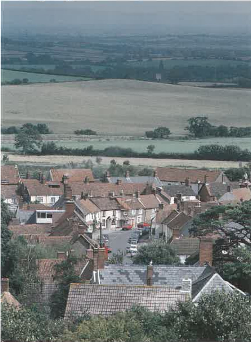
Landscape context. There is a need to pay special attention to the preservation or enhancement of character and appearance, not just of historic buildings. It should also be a material factor in assessing development proposals outside conservation areas which may reflect its setting or views into or out of the area.
