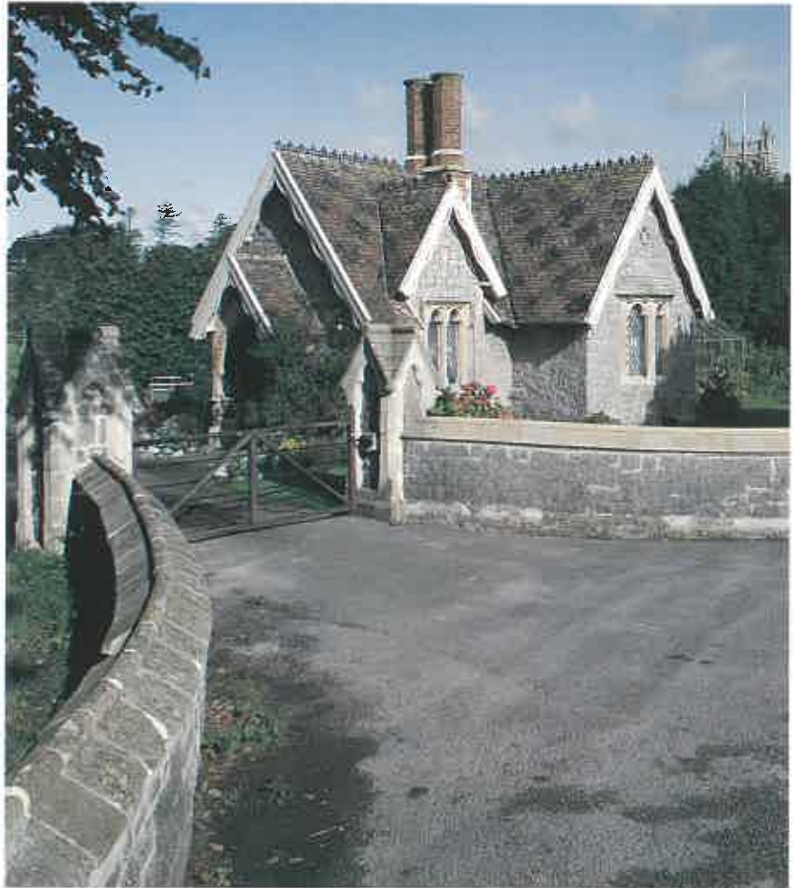
The Stephenson gothic legacy as epitomised in the rich detailing of the Manor Lodge. The roof is of plain and "fishtail" tiles in a diaper pattern with crested ridge. The splayed rubble walling and dressed stone cross-gabled caps to the piers echo the extravagant gabling to the lodge.
