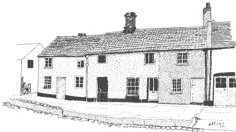
Originally divided from a 16th century cross passage house, Nos. 20, 22 and 24 Castle Street (south side) represent three simple cottages and were listed in 1985 as part of the national re-survey. The statutory protection of such buildings recognises the enormous contribution of vernacular buildings to the character of historic villages. No. 24 (right) was extensively repaired with grant aid from the District Council in 1987 thus helping to reinforce investment confidence in the conservation area.
