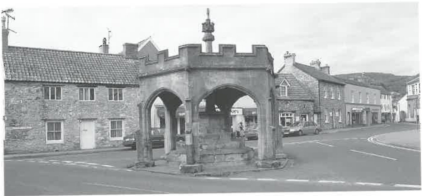
Cheddar market cross, one of Somerset's magnificent remaining monuments of its kind. Originally a preaching cross it was later surrounded (probably in the 17th century) by a hexagonal structure with open arches providing a dry market for itinerant merchants. Dominant in the street scene and the focus of the conservation area, the structure is so obviously physically vulnerable to traffic.
